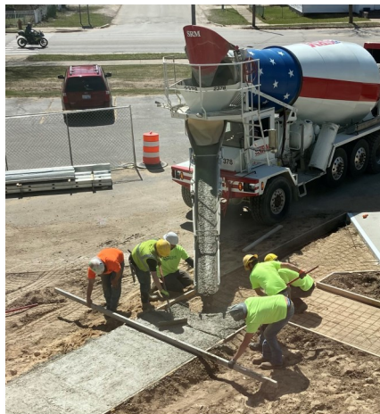
Concrete sidewalks being poured.
