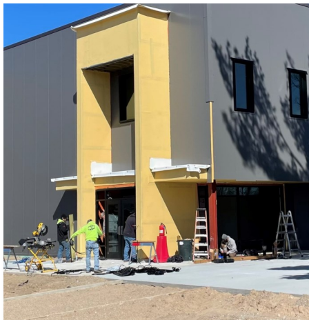
Work on new public entry
